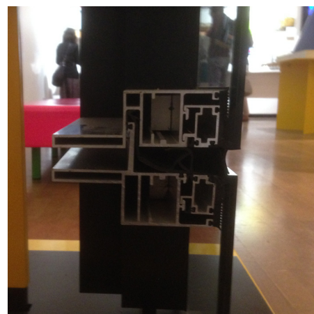
Example of another the prefabricated Steel component and joint to the window panes. Photo by Brandon Whitwell-Mak, taken at the Richard Rogers RA: Inside Out exhibition
