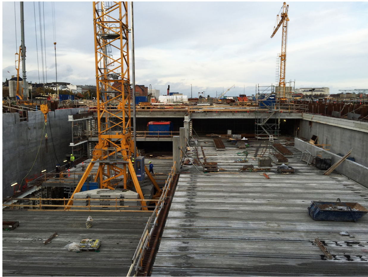
Carpark in construction
