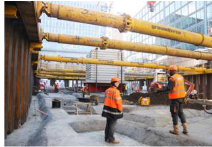
Example of modular propping for the building of a basement
