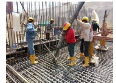
site cast concrete slab
