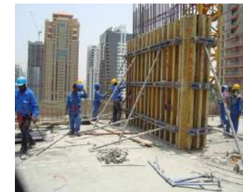
site cast columns of reinforced concrete in sheet piles
