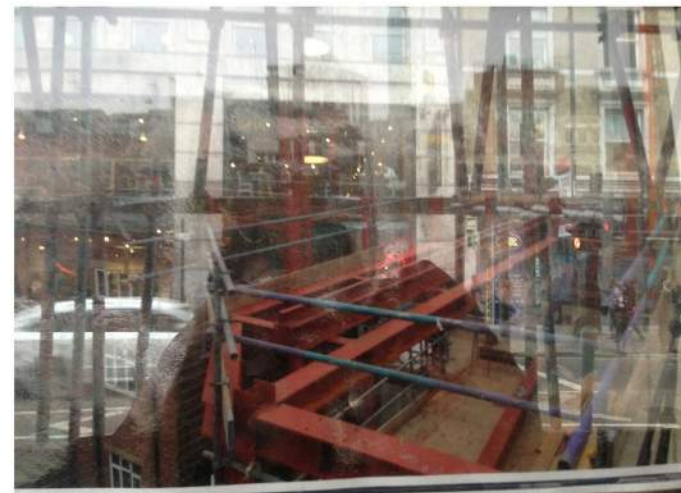
Above: Steel construction on the construction site
