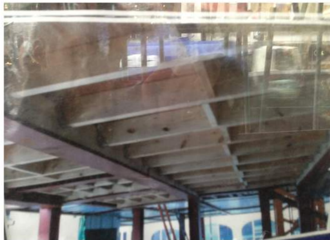
Above: Substring construction on the construction site
