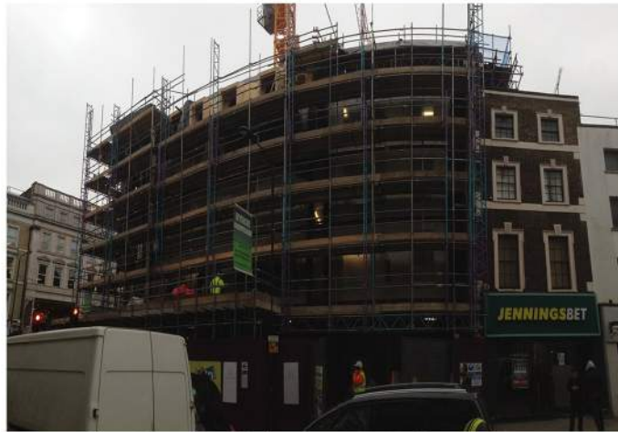
Above: Present views for the construction site: from Goodge street
