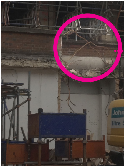
Morwell Street Construction Site
