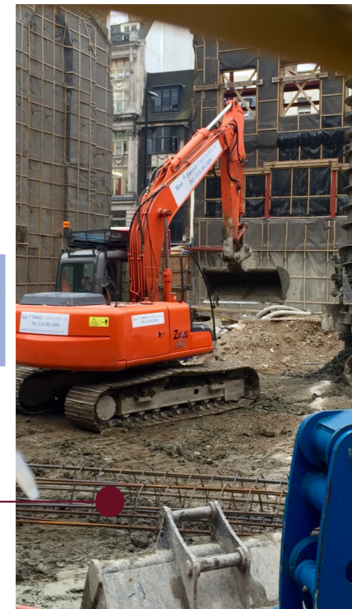
Steel spiral wire frame that acts as reinforcement for future concrete column. Reinforced columns are cast on site.
