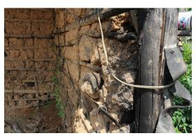
Mud walls are constructed using clay dug up on site from the process of mining gems. Growing plants brings an unintentional expressive quality to the faced
