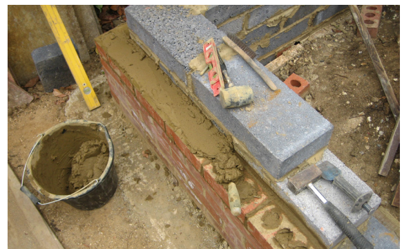
brick and mortar laying
