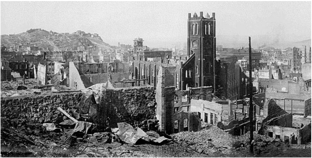
brick structures are destroyed during earthquake
