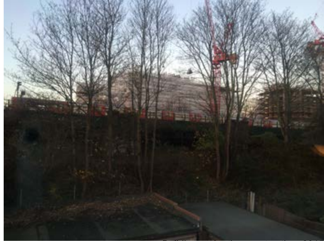
Building under the construction, 2015
