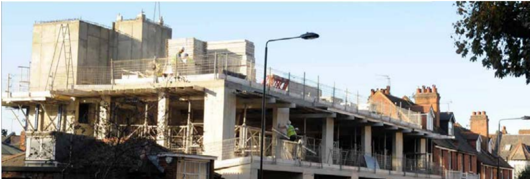
Building under the construction, 2015
