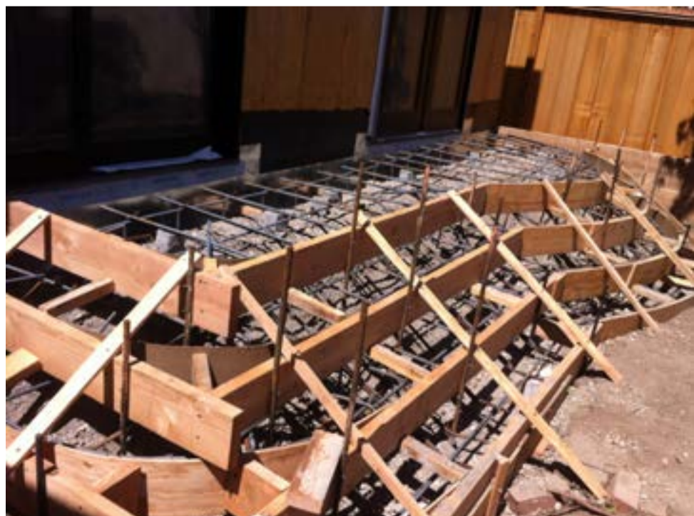
Curve concrete formwork
