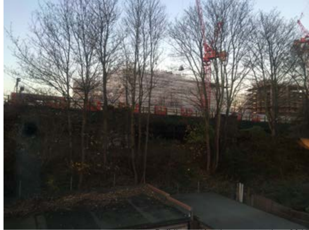
Building under the construction, 2015
