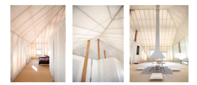
The concrete slab retains heat from underfloor systems and by way of the central hearth. The walls and roof are composed of three layers of materials: polyester fabric, an insulating layer made from recycled PET bottles and a removable inner curtain made from glass fiber. The transparent structure was designed for "a life surrounded by natural light."
