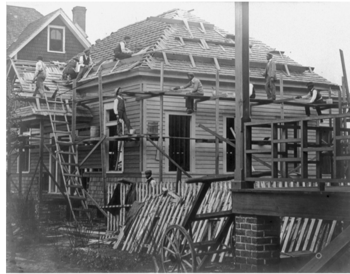
Supporting from the ground
