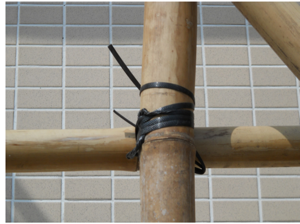
Bamboo structure with strings or ropes tied them together
