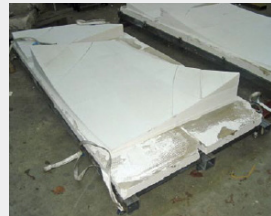
Large moulds are milled from cellular concrete and placed in the furnace in 700 Celsius degree
