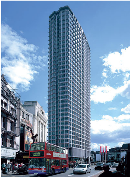
Centre Point Building
