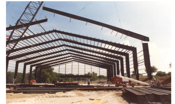
Conventional Steel Fabrication
