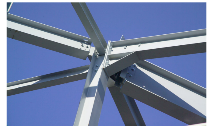
Bolted Steel Construction
