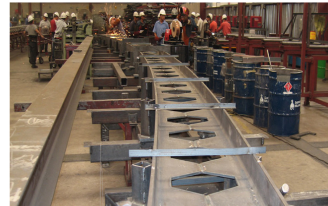
Conventional Steel Fabrication
