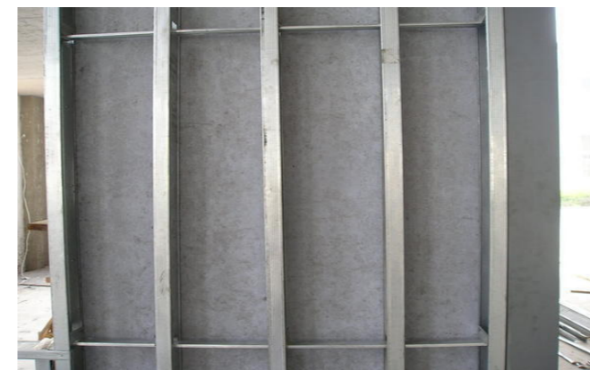
Light Gauge Steel Construction
