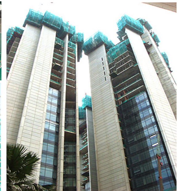
Perfect fare faced concrete through precast panels.
