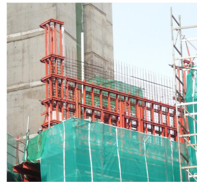
Installation of the precast panel
