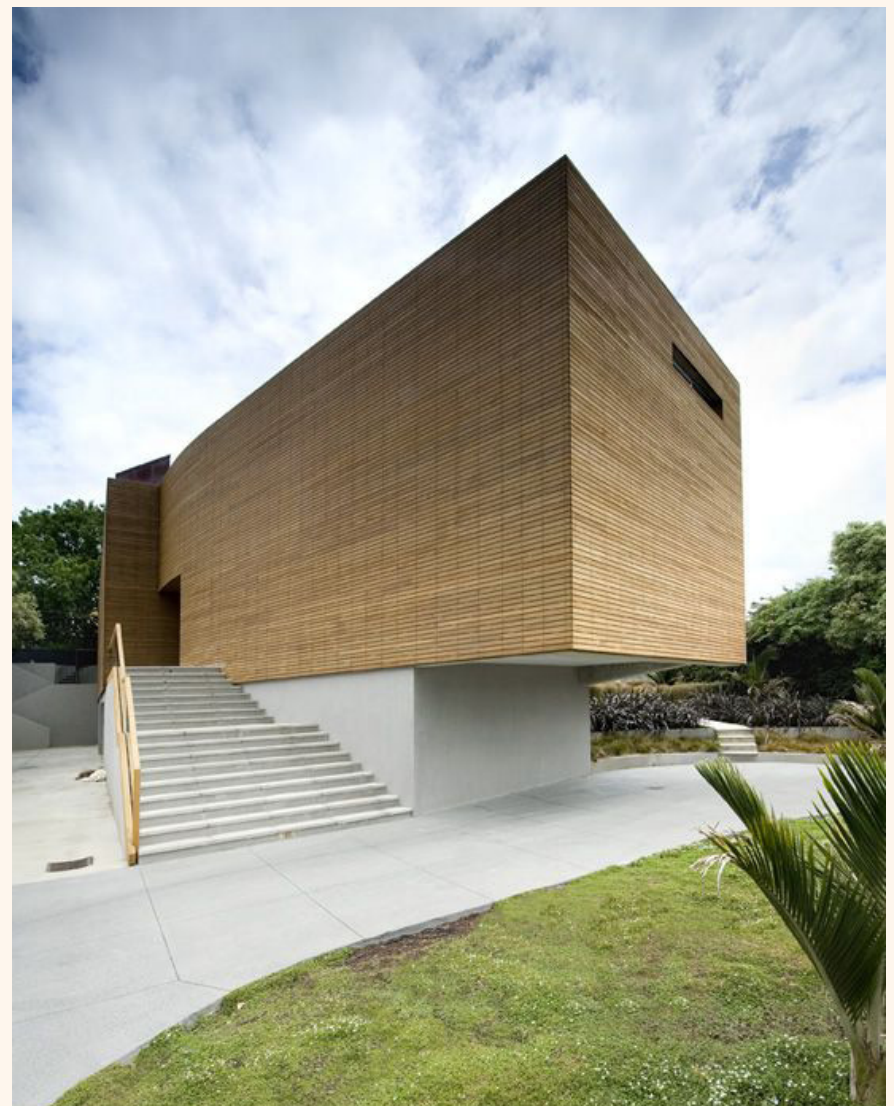
Big House by Glamuzina Paterson Architects
