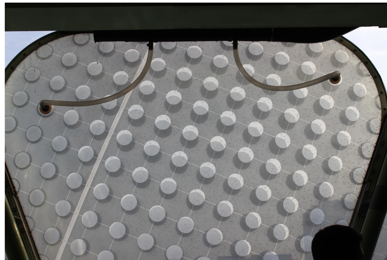
Image 6 The ETFE cushion is connected to sensors that control its inflation and deflation throughout the day.
