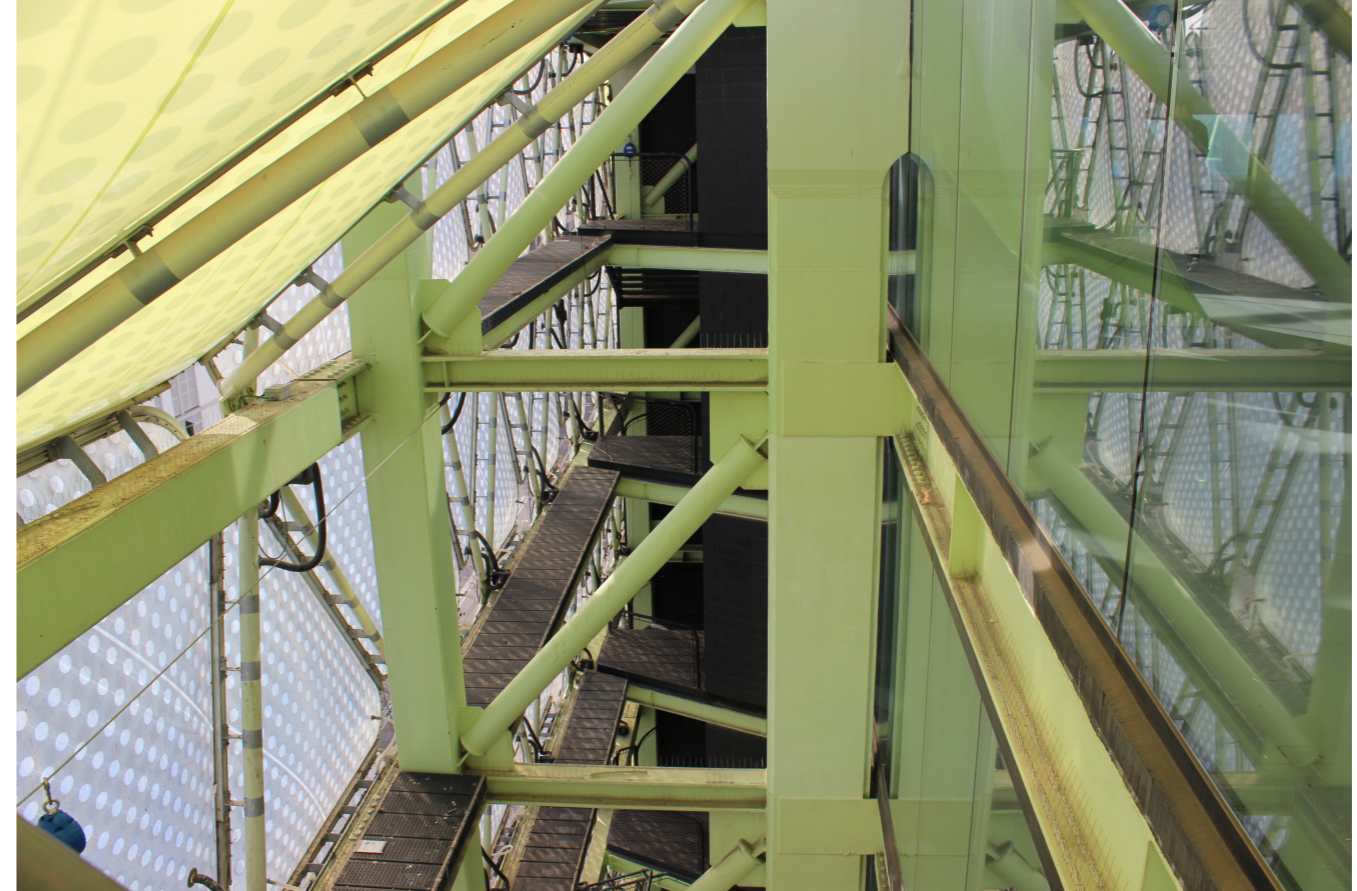
Image 3 Inside the Envelope: The ETFE cushion façade a separate entity, completely disconnected from the inner membrane of the building.
