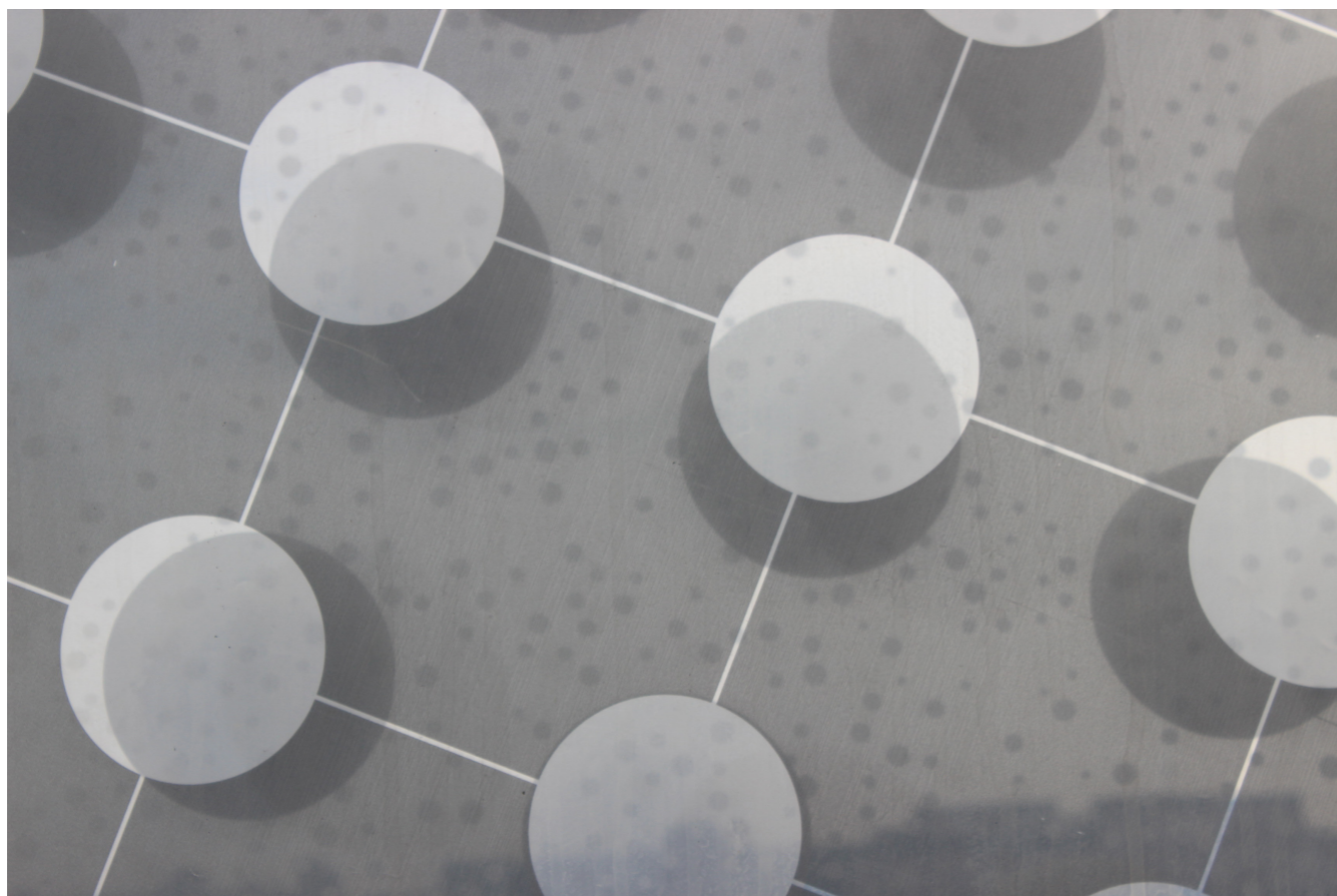
Image 5 Close-up of Photo Voltaic circles that enhance the performance of the ETFE cushion.
