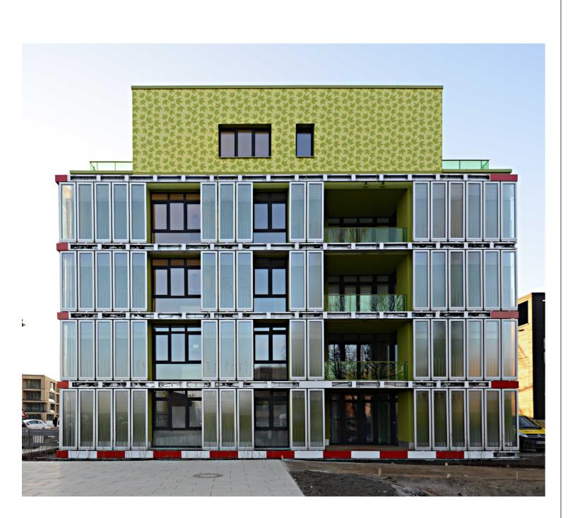
The solar leaf facade was first tested and insalled on a large scale building in the BIQ house at the IBA in Hamburg in 2013. In total, 129 bioreactors have been installed on the south-west and south-east faces of the four-storey residential building to form a secondary façade.
