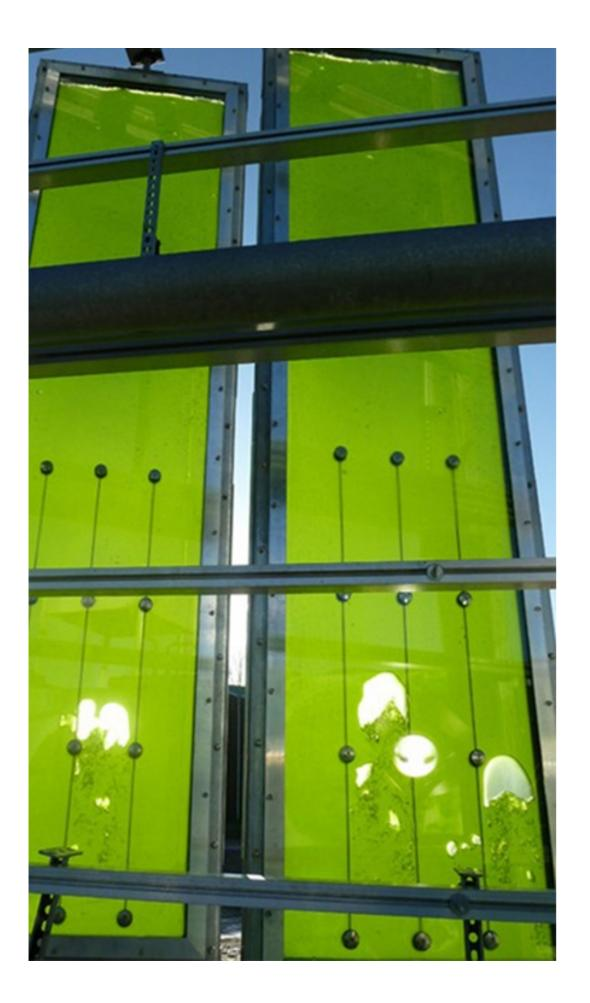
The facade is built from integrated photo-bioreactors. It aims to provide shade and a renewable fuel source for the experimental apartment. This revolutionary solution has multiple advantages and functions. It provides dynamic shading, thermal insulation and noise abatement,
