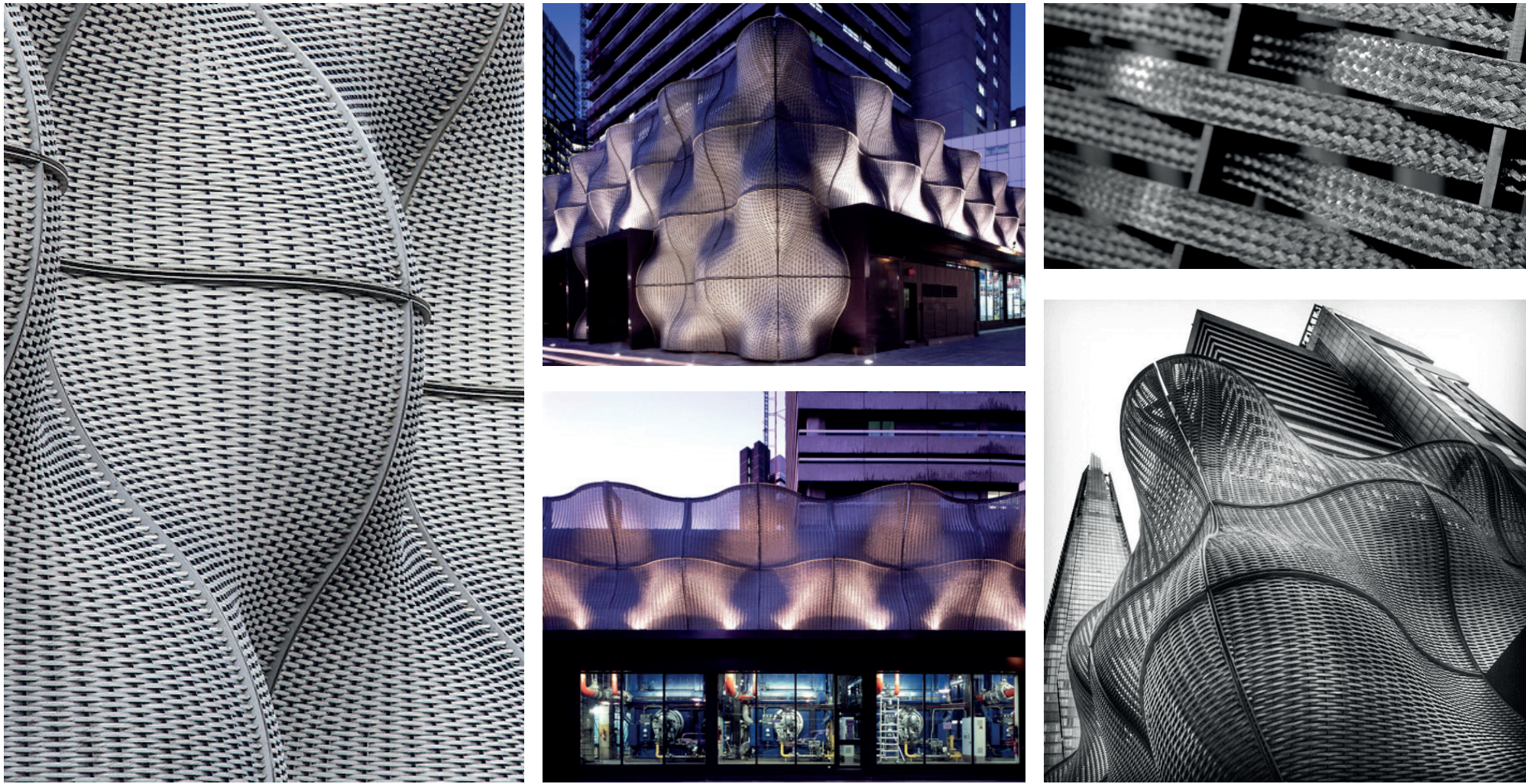
Thomas Heatherwick has completed Boiler Suit, an undulating facade of woven steel panels encasing the boiler house at Guy's Hospital in London. At the centre of the scheme is the Boiler Suit, a unique façade designed to encase the boiler house which powers Guy's Hospital. The Boiler Suit is made up of 108 undulating tiles of woven stainless steel braid and is illuminated at night to provide a distinctive welcoming beacon for staff and visitors arriving at hospital in the dark.
