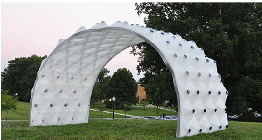
Thermoplastic Welding Technology and Dohle Extrusion Fabrication: Robotic Fabrication Lab (RFAB)
